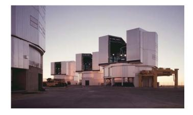
**FIGURE 6.26** The Very Large Telescope (VLT), operated by ESO in Chile. Movable auxiliary telescopes allow the four large telescopes to operate as an optical interferometer.
